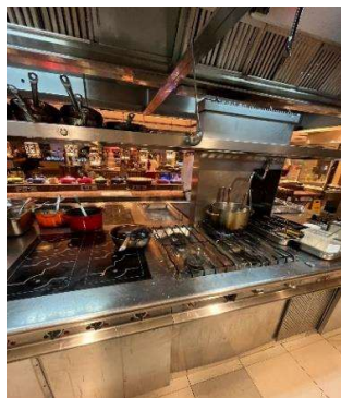
Figure 3. 15 In Room Dining Hot Kitchen
