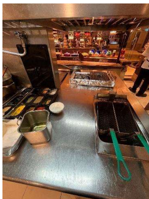
Figure 3. 16 In Room Dining Hot Kitchen
