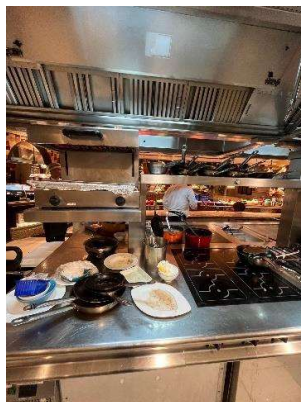
Figure 3. 14 In Room Dining Hot Kitchen
