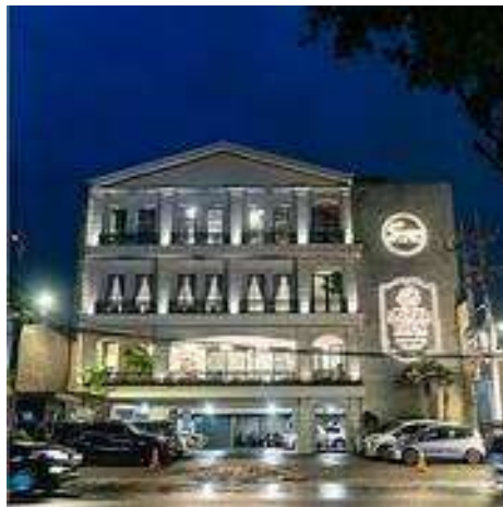
Figure 1. 1 Latar Ijen Resto & Coffee shop
