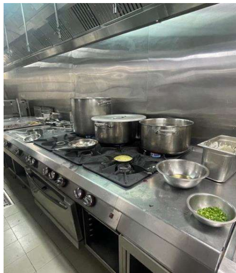
Figure 3. 80. Japan kitchen inside
