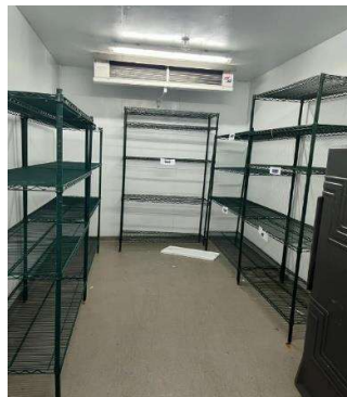
Figure 3. 41 Inside meat and Fish Chiller for all Outlet
