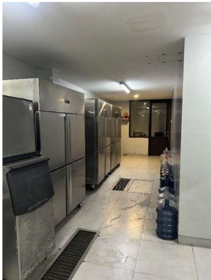
Figure 3. 13 Freezer & Chiller Area
