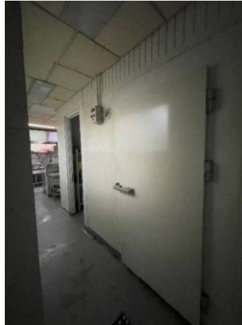
Figure 3.15 Kitchen Dry Storage and Walk-in Chiller
