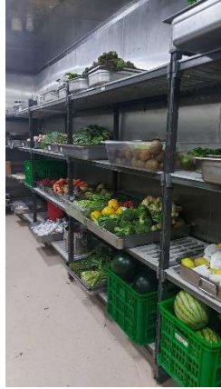
Figure 3. 51 Walk In Chiller
