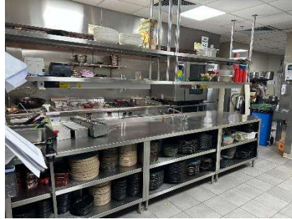
Figure 3. 46 Western Section Kitchen
