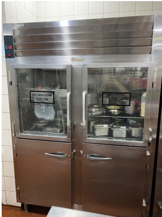
Figure 3. 25 Pavilion chiller (Personal Documentation,2023)
