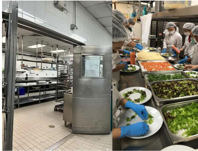
Figure 34. BCC Cold Kitchen
