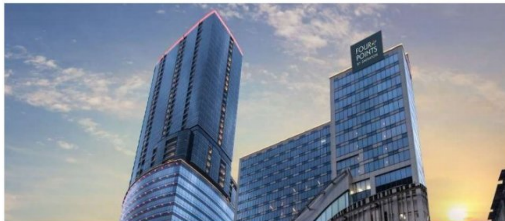
Figure 3. Four Points by Sheraton Tower
