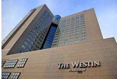
Picture 1 The Westin Hotel in Warsawa, Polandia
