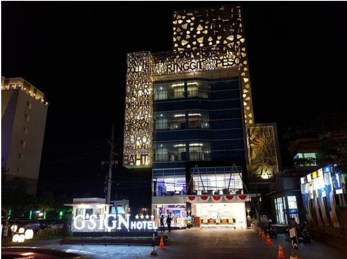
Picture 2. G'SIGN Hotel front view (G'SIGN HOTEL Gallery, 2018)
