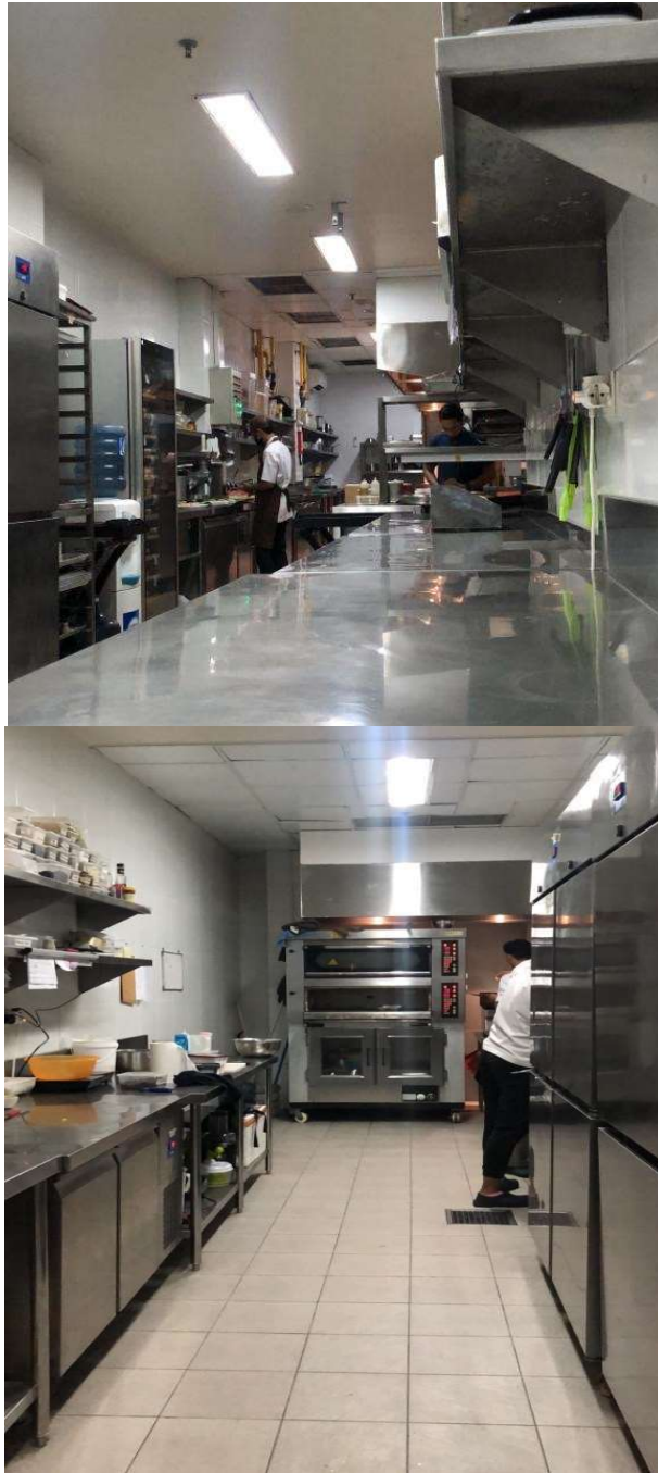
Picture 22. Kanvaz Patisserie (Tearoom) Kitchen
