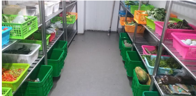
Figure A9 Clean Chiller
